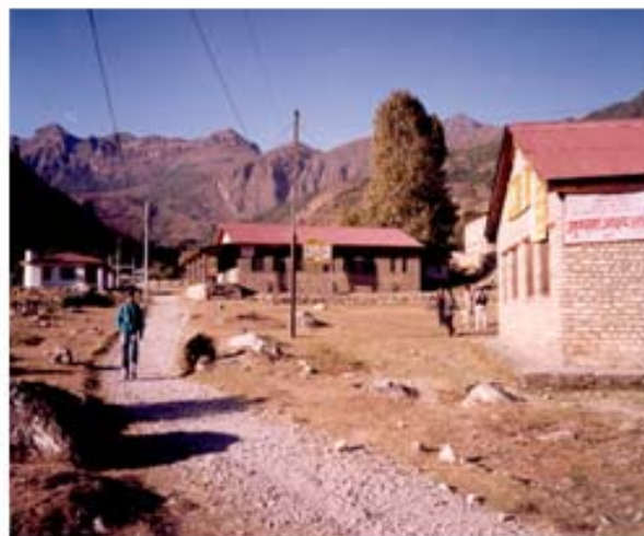
View of existing blocks and new construction site
